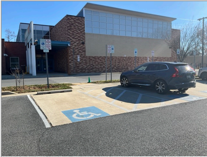
OVERVIEW OF ACCESSIBLE PARKING AREA
