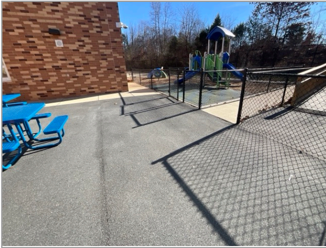
ACCESSIBLE ROUTE TO PLAYGROUND
