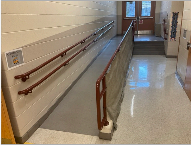
ACCESSIBLE INTERIOR RAMP
